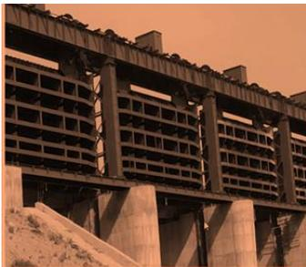
**Fig.2. Vertical lift slide gates (courtesy- Walchand Institute of Technology, Solapur) [4].**
