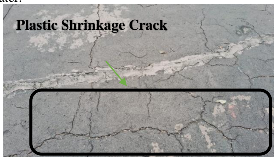
Fig. 4- Plastic shrinkage crack
